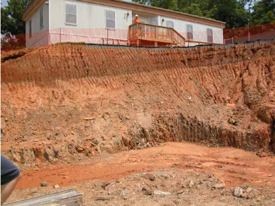
Due to the difference in site grading between the school level and the field level, there would be significant site excavation for a new addition should it be at the same floor level as the school. The site is known to contain some ledge which will have a cost impact on the construction.
